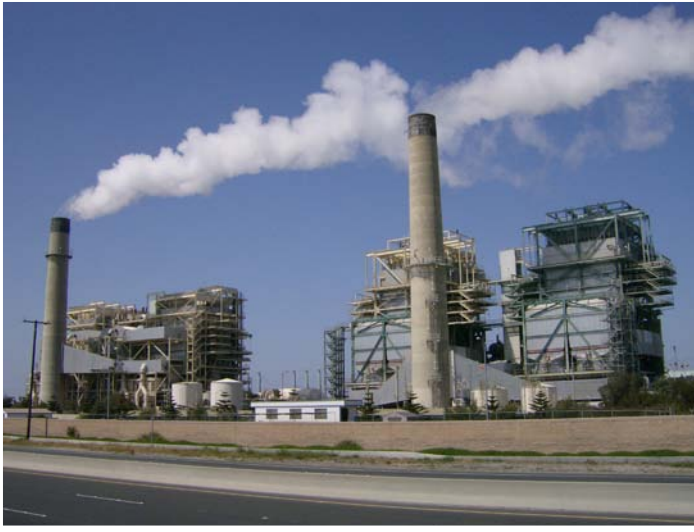
Seawater desalination plant.
